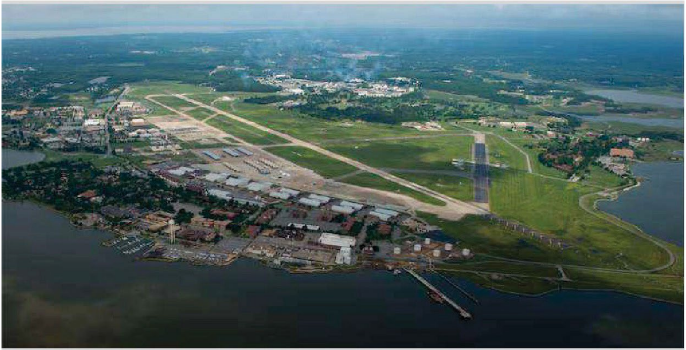
Aerial image of Joint Base Langley-Eustis. (Source: DOD 2024)
