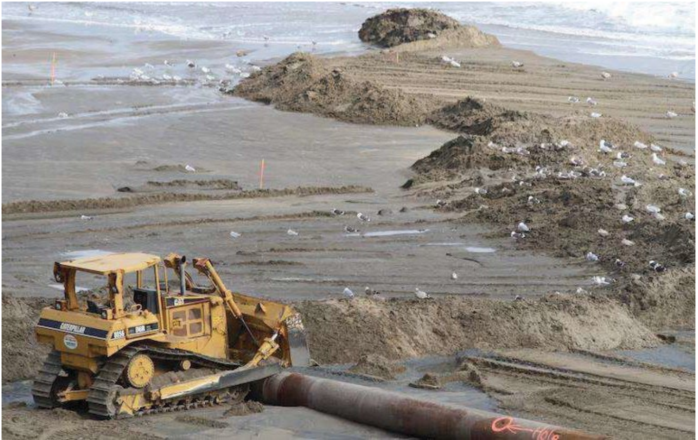
A beach nourishment project underway at Virginia Beach in 2013. (Source: USACE)
